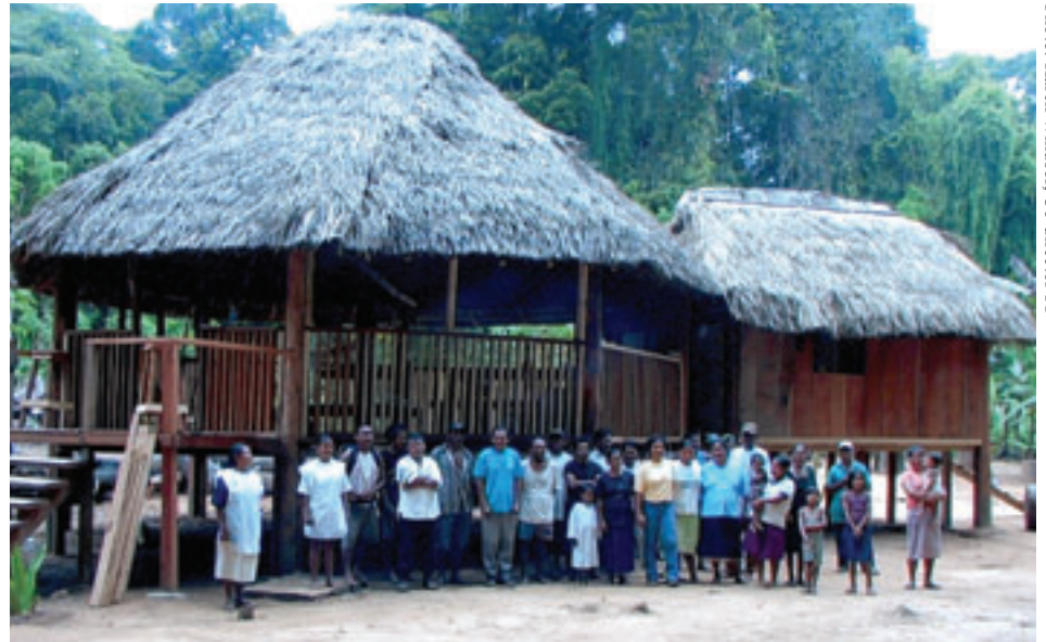
In this photo are those who took the courageous step into their own future. The lodge complex has been built entirely by labor donated by these wonderful people. Entire families have moved onto the site while work is completed.
